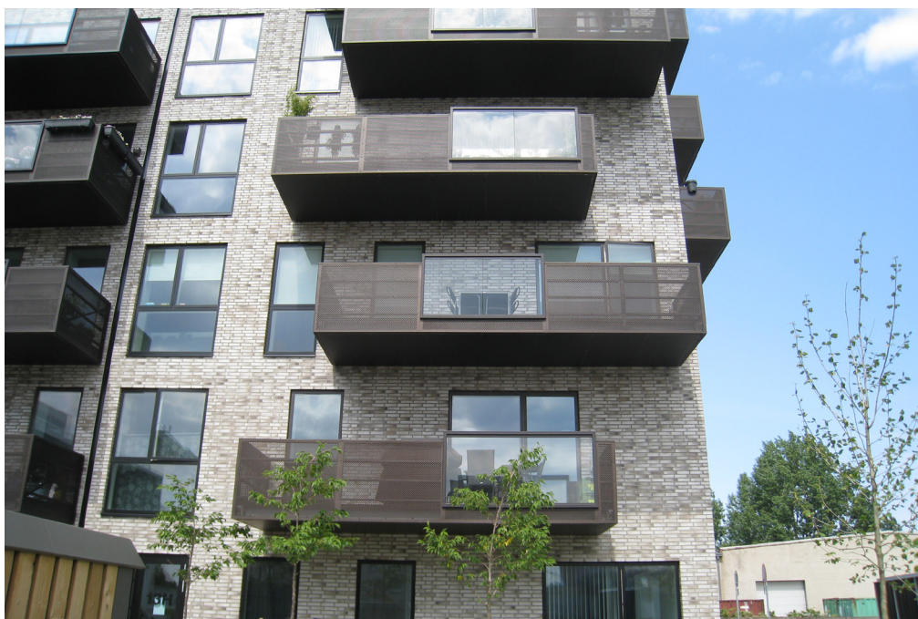
Perforerede aluminium plader, Anodiseret. Perforering langhuller LR8 x 25, deling 30 x 32 mm
